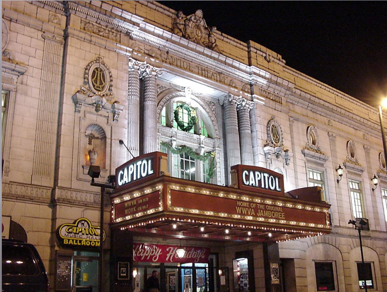
Wheeling National Heritage Area, WV
